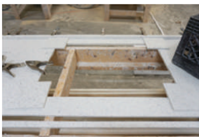
Underside of cooktop cutout with reinforcing blocks in place
