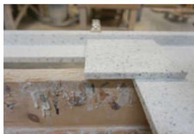
Close-up of reinforcing block in place
