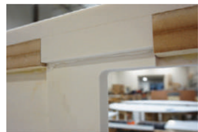
View of reinforcing block after finishing
