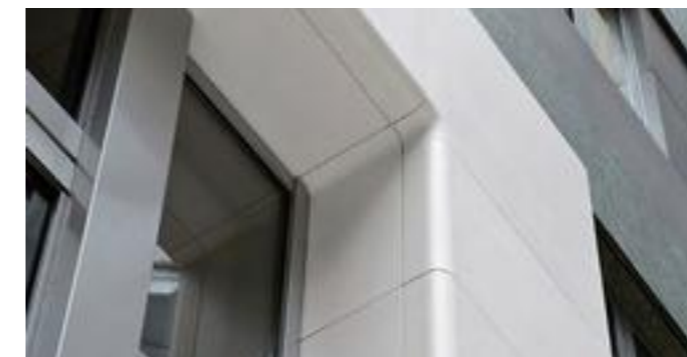
One of the most important features when using HIMACS on a facade is its ability to create round corners.
